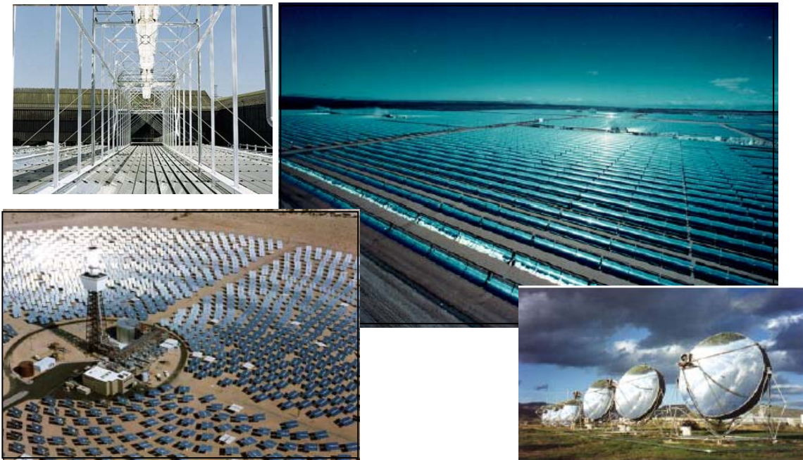
Fig. 6: Different kinds of solar thermal power plants from the upper left corner clockwise: Linear Fresnel project (Solarmundo), Parabolic Trough ‘SEGS’ (California, PSI), Paraboloid Dish Sterling (SBP), Tower System project ‘Solar Two’ (California, SNL) (Source: DLR, 2005; Trieb & Milow, 2000).
