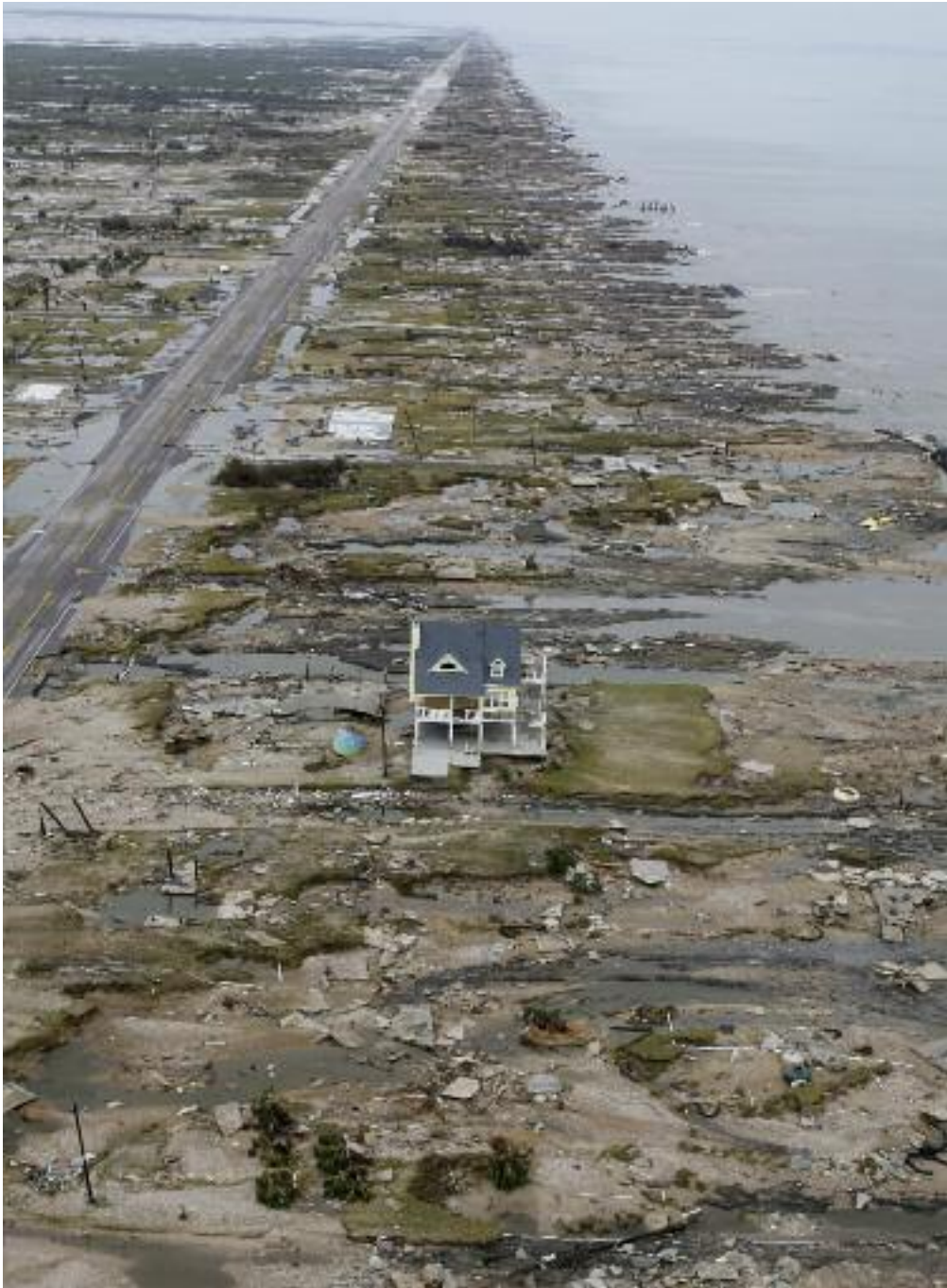
Hurricane Katrina, which devastated a large part of the Mexican Gulf coast of the USA in 2005, caused tremendous damage and suffering for residents. The photo shows part of New Orleans. (Photo: Scanpix)
